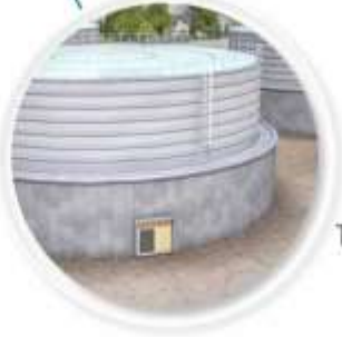
Tank Ring Walls
