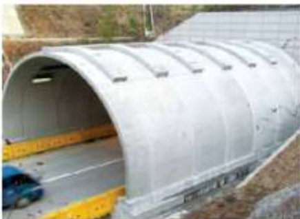
Tunnel extension - Hyeongok (South Korea)
