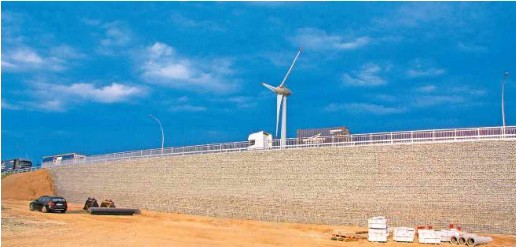
Retaining Walls in Altenwerder
