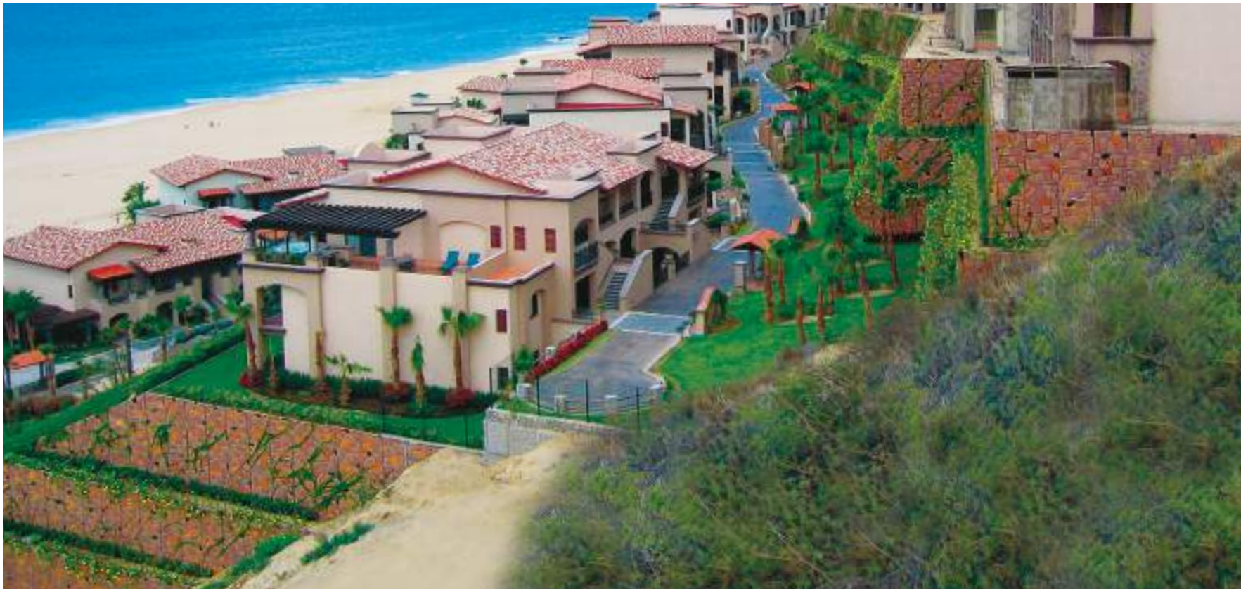
Pueblo Bonito Hotel Cabo San Lucas, Baja California, Mexico ▶
