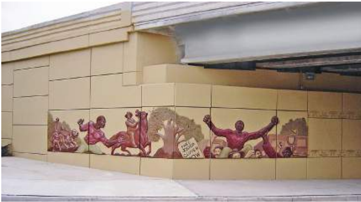
Marquette Interchange Milwaukee, Wisconsin, USA ▶
