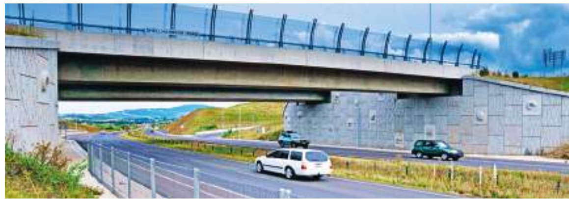
Oak Flats Interchange, South Coast
