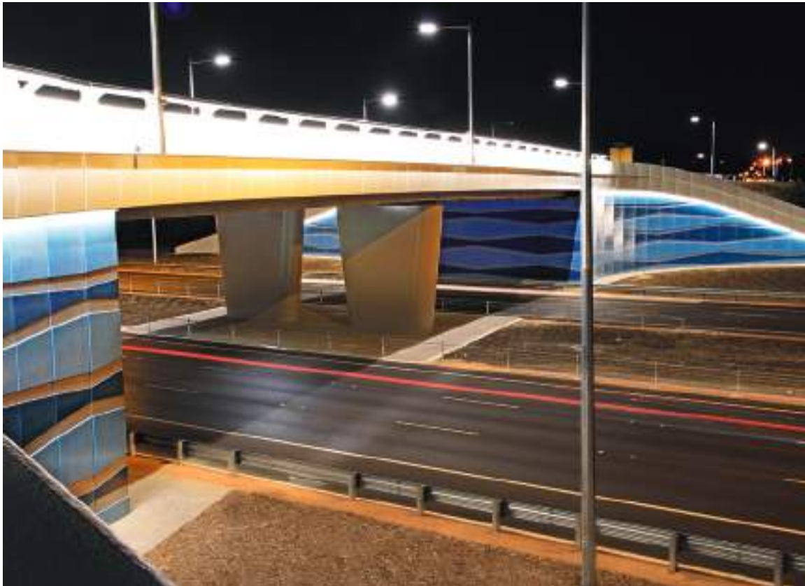
Tonkin Highway / Dunreath Drive Interchange, Gateway Western Australia Perth, Western Australia, Australia ▶
