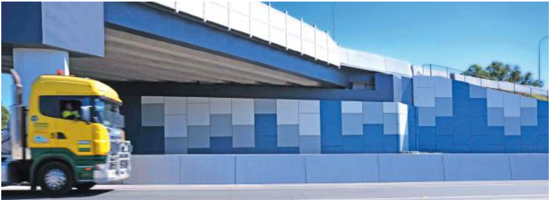
Darra to Springfield Transport Corridor Brisbane, Queensland, Australia ▶
