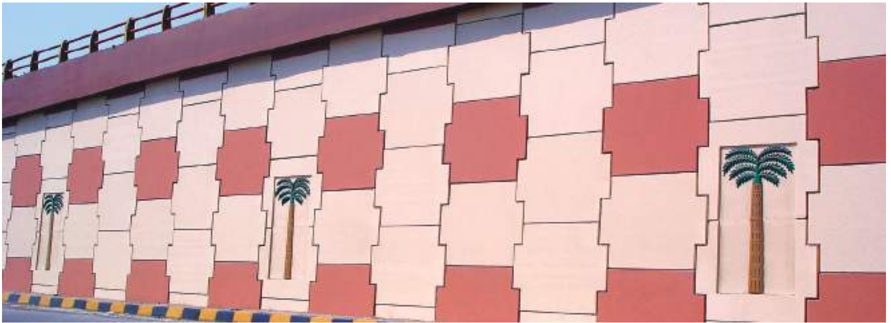
Navghar Flyover, Mumbai International Airport Mumbai, India ▶
