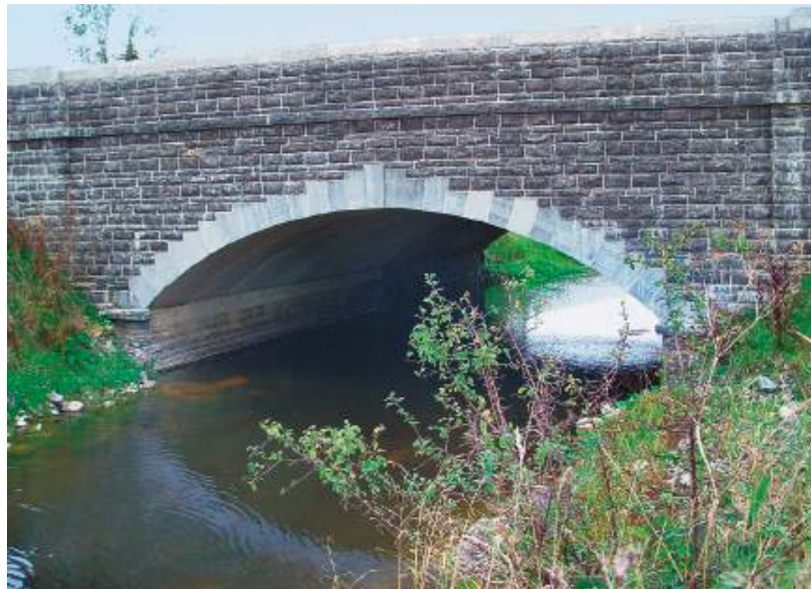
Scramoge Bridge National Road N5, Roscommon County ◀ Scramoge to Cloonmore, Ireland
