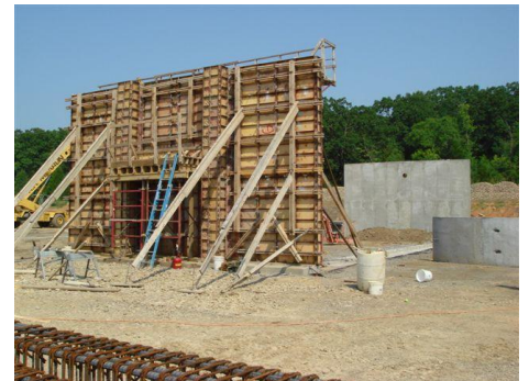
FRONT AND REAR WALLS BEING READIED FOR ARCHES
