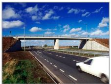
The Highways Agency required a temporary solution to address safety issues at a problematic crossroads on the A1 trunk road. The proposed structure was intended to be used for a minimum of 10 years, with the possibility of the life-span being extended. The structure needed to be capable of being dismantled and re-used elsewhere. In order to minimise disruption to the adjacent carriageway, speed of construction was a key factor in selecting the preferred solution.
