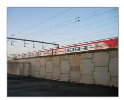
Network Rail's £350 million Trent Valley Four Tracking Project increased capacity on the West Coast Main Line, doubling the tracks from two to four along a 12 mile stretch of railway between Armitage with Handsacre and Tamworth and removing a major bottleneck.
