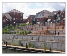
Although in an urban setting, the site planning requirements dictated an environmentally sympathetic face to the canal. In addition, the unknown condition of the canal edge would not allow heavy structures to be situated close to the watercourse. The structures also had to allow for a terraced garden style layout and ease of access to the canal side for the property owners.
