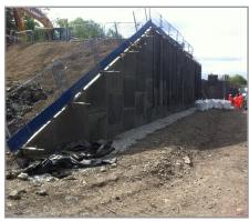
Reinforced Earth Co. Ltd (RECo) was employed to design and supply the components for Muller Road Reinforced Earth retaining wall, as part of Network Rail's upgrade plan to increase the rail capacity from two tracks to four tracks between Dr Day's junction to Filton Abbey Wood, to the north of Bristol.
