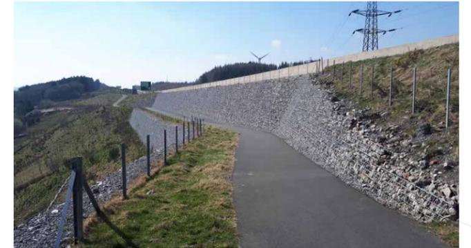
On the other side of the new road a Reinforced Earth steep slope with a stone finish was used to provide the support to the carriageway alongside a pedestrian route.
