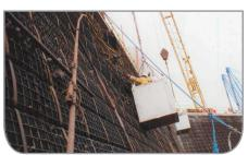
Reinforced Earth<sup>™</sup> wire mesh facing system, used on the Second Severn Crossing, won a British Construction Industry Award.
