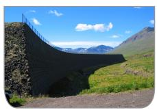
The project involved the construction of avalanche defences at Neskaupstaður Iceland. The defences comprised a 14m high catching earth dam and 13 No. 10m high breaking earth mounds (splitters) in the run out zone of snow avalanches. The defences formed the first phase of avalanche protection works to the town of Neskaupstaður on the east coast of Iceland.
