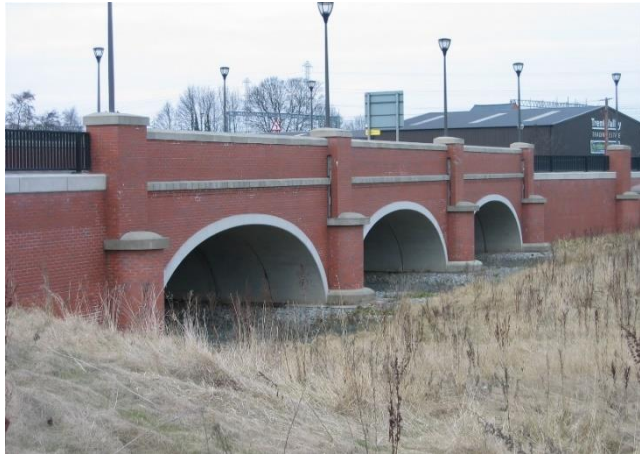
Flood protection with precast arches
