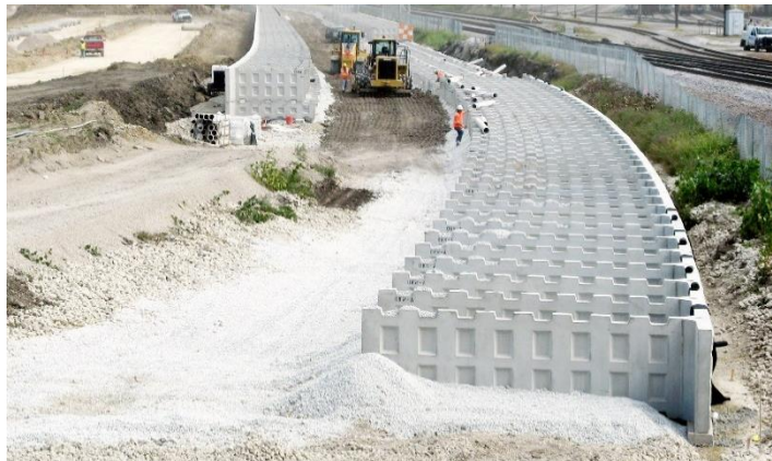
T-Wall rail embankment back to back walls
