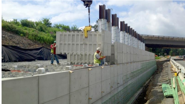
T-Wall bridge abutment
